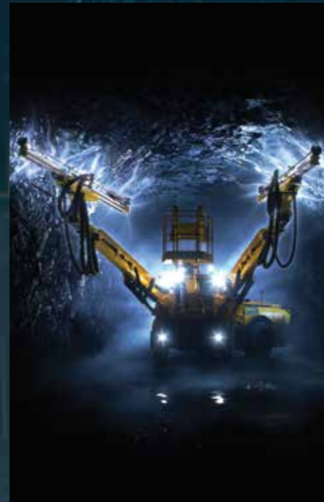
Underground civil engineering
